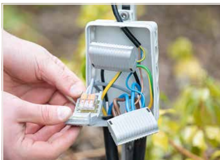
Connecting a bollard light
